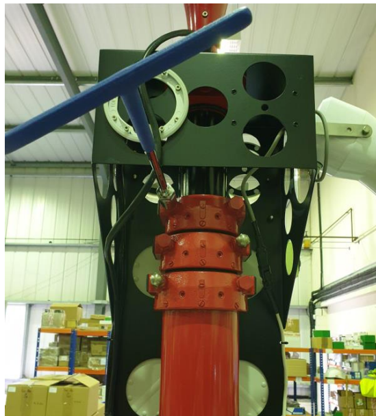
Figure 15 - Lowering the Mast Step 4
