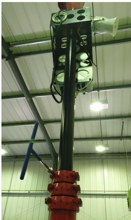
Figure 13 - Lowering the Mast Step 2
